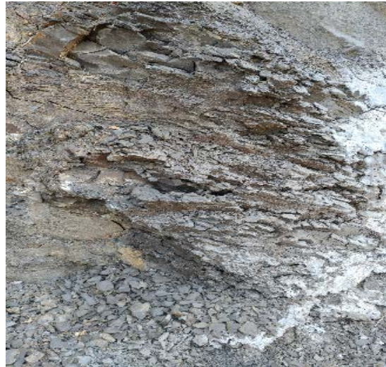
Fig. 2. Condition of clay shale in Sentul City that has been exposed
